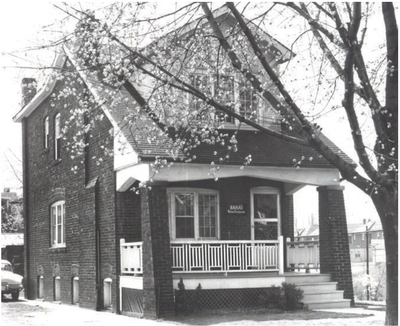
15 Lola Road in Toronto, Ont., which served as the Bahá'í National Centre from 1957 to 1969, pictured in 1963.
