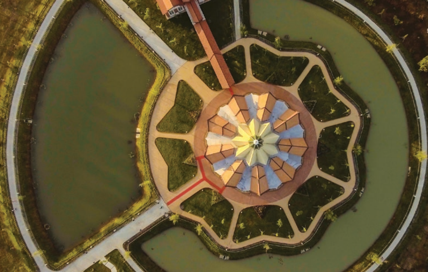
Aerial view of the local Bahá'í House of Worship in Battambang, Cambodia. Photo: Bahá'í International Community
